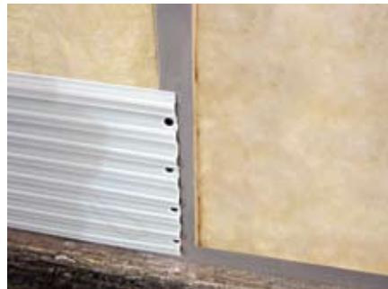
2 #1033 - Primary Insulator, fastened horizontally to the studs
